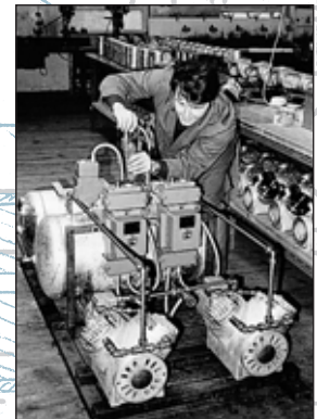
Compressor plant being assembled (1968)
